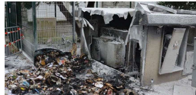
Lorient (Morbihan), 1 st July: from rubbish bin to electric substation...
