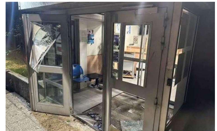
Kremlin-Bicêtre (Val-de-Marne), night of 29/30 th : entrance of the pig shop
